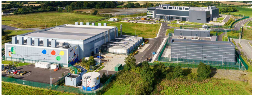
One of Google's data centers (Dublin, Ireland)
